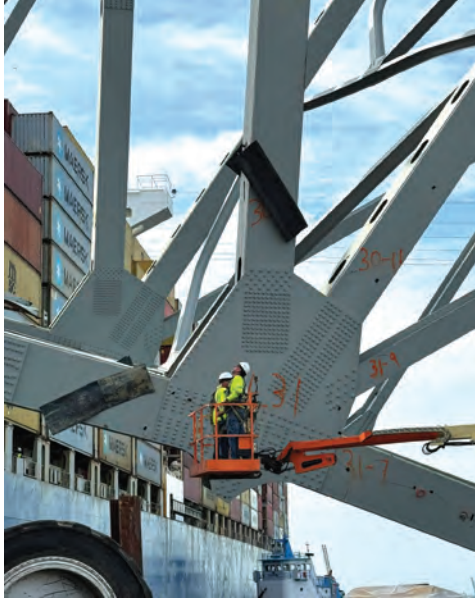
Preparing for the demolition involved precision torch cutting for subsequent placement of explosives.
