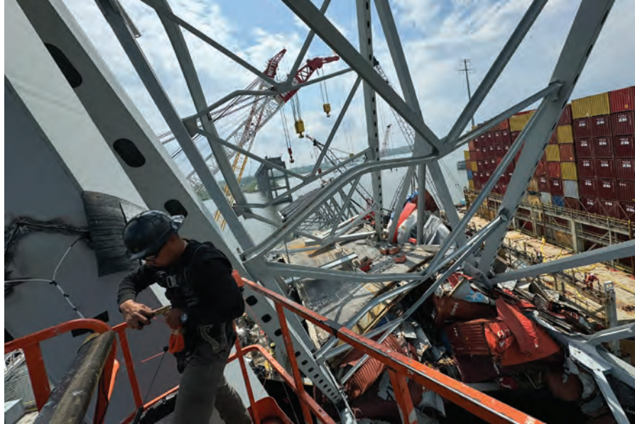
Preparing for the demolition involved precision torch cutting for subsequent placement of explosives.
