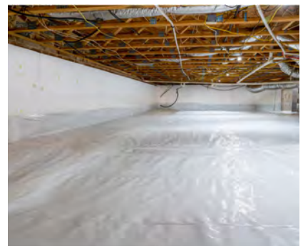
Left: Before encapsulation, crawlspaces can have issues with moisture, pests and inefficient insulation. Right: A properly encapsulated crawlspace can solve those problems. Tip: When installing poly liners, seams should overlap by at least 12 inches. White poly is often sealed with white tape to maximize the visual impact.
