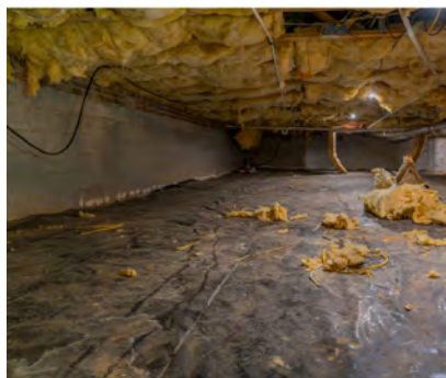
Left: Before encapsulation, crawlspaces can have issues with moisture, pests and inefficient insulation. Right: A properly encapsulated crawlspace can solve those problems. Tip: When installing poly liners, seams should overlap by at least 12 inches. White poly is often sealed with white tape to maximize the visual impact.
