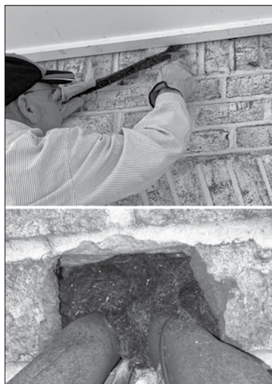
Plugging holes with products such as Xcluder® rodentproofing fabric effectively exclude rodents from entering openings in foundation walls until permanent construction changes can be made.
